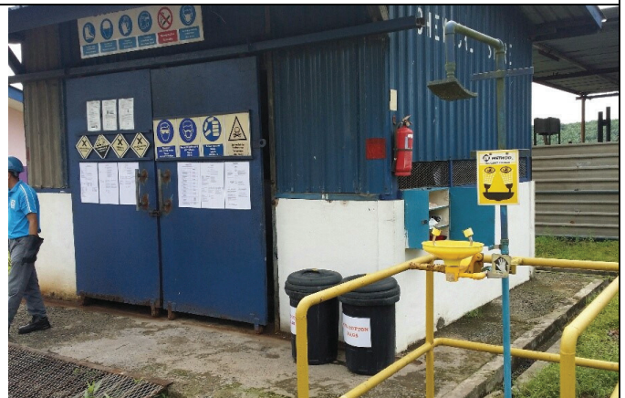
Chemical store and shower/eye wash facility.
